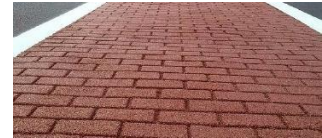
Figure 3. GeoBondX creates durable stamped crosswalks
