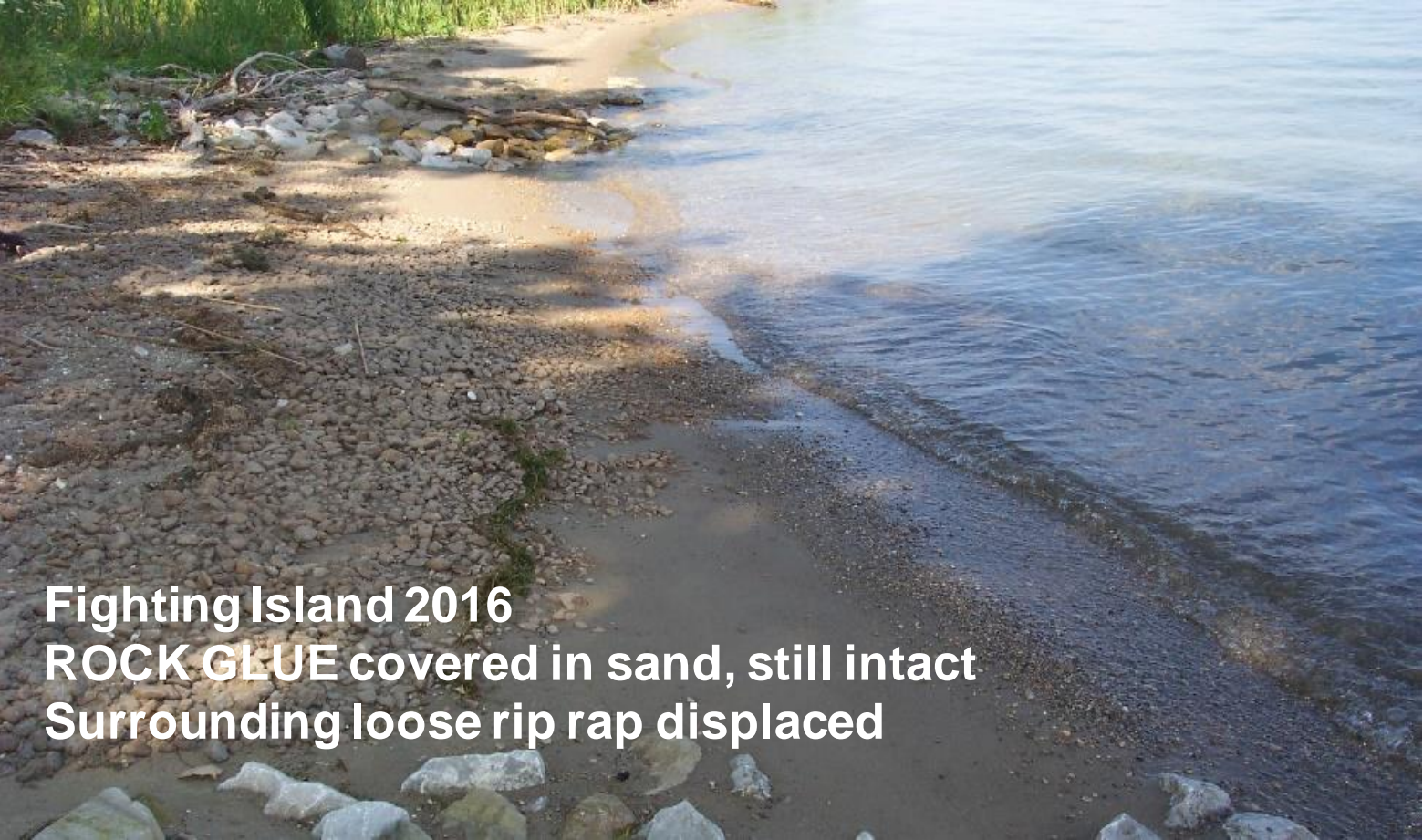
Installation: September 2007 First North American pilot project PU in Coastal Protection
