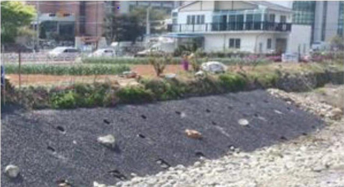
(a) During construction
